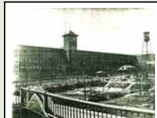
Loray Mill with playground
