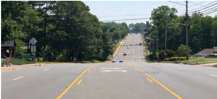
FIGURE 36: TYPICAL CONDITIONS ON GARRISON BOULEVARD
