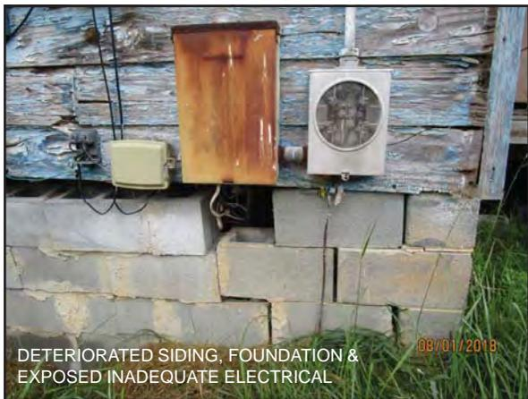
DETERIORATED SIDING, FOUNDATION & EXPOSED INADEQUATE ELECTRICAL 08/01/2018
