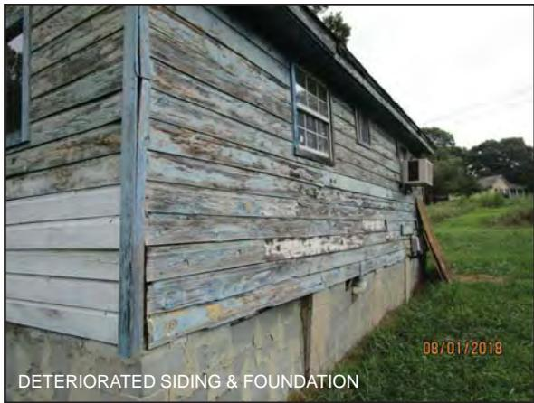
DETERIORATED SIDING & FOUNDATION 08/01/2018
