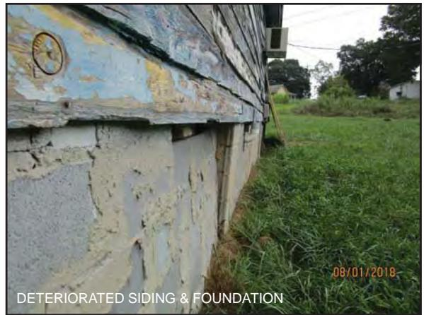
DETERIORATED SIDING & FOUNDATION 08/01/2018
