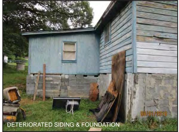
DETERIORATED SIDING & FOUNDATION 08/01/2018
